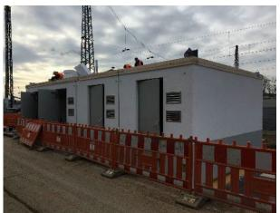
A modular building for a track-field concentrator (GFK)
