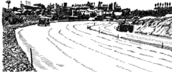
PREPARING THE ROAD BASE
