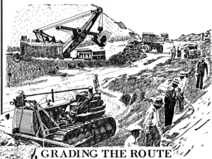
GRADING THE ROUTE
