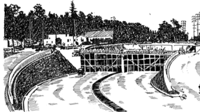
INSTALLING CURBS & GUTTERS
